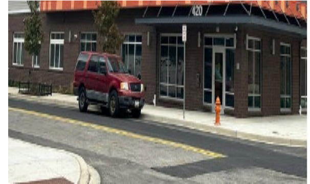
New Sidewalk and Road Infrastructure at Somerset
