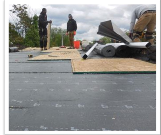
Vacant Property Roof Stabilization
