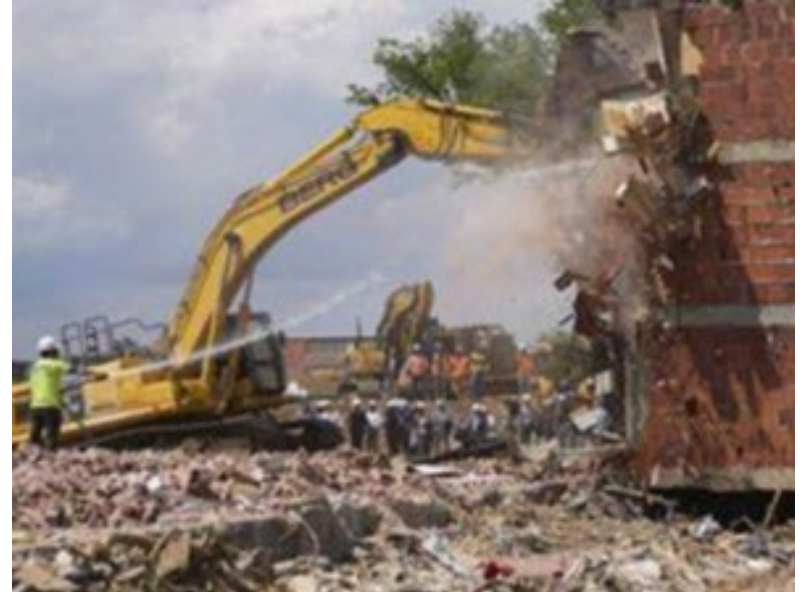
Demolition at Perkins
