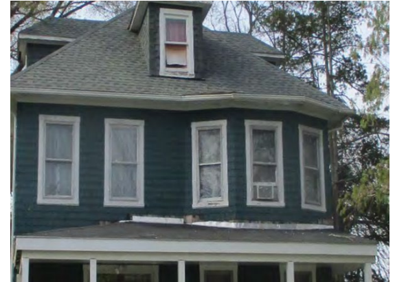
Before & After Window Replacement Done as part of the Lead Hazard Reduction Program
